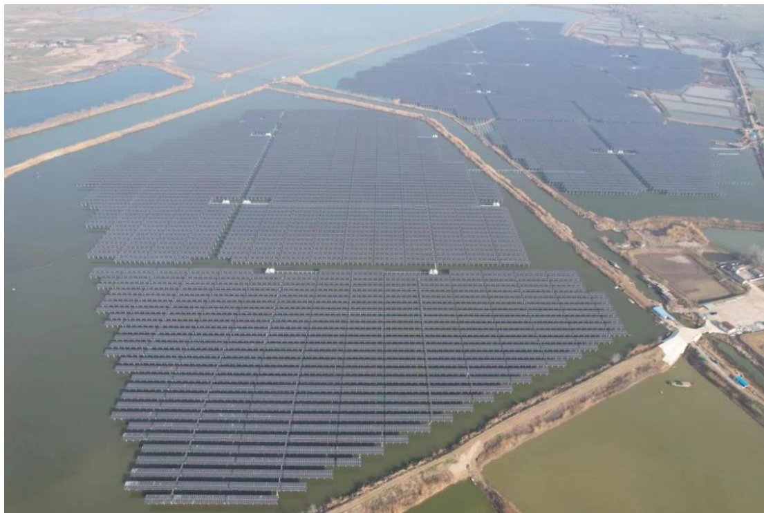
The 300MW Fishery-PV Integration power plant project by a PV power generation company
